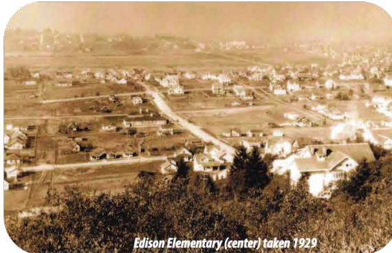
Edison Elementary (center) taken 1929
